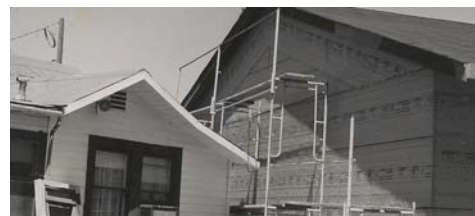
The sanctuary being built next to the cottage
